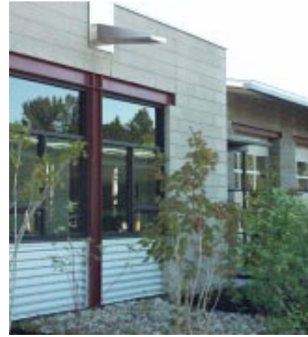
Roof runoff is directed to scupper gardens where the water is filtered naturally.
