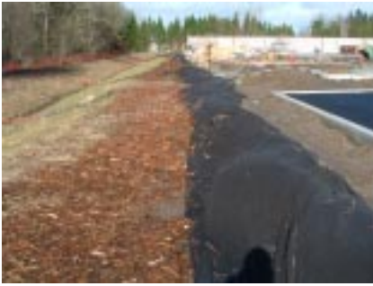
Woody debris was wrapped in filter fabric to create rows of protective barrier during construction. Afterward, the swale was reshaped and planted with native plants shown to the right.
