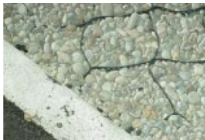
Reinforced gravel in the storage yard.
