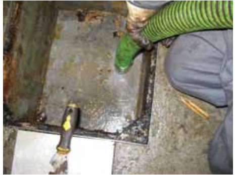
Oversee contractors for complete, correct service.
